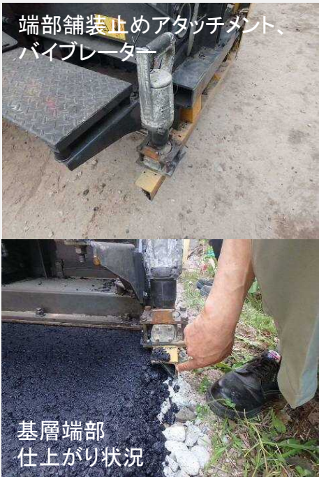
①基層の無型枠施工
