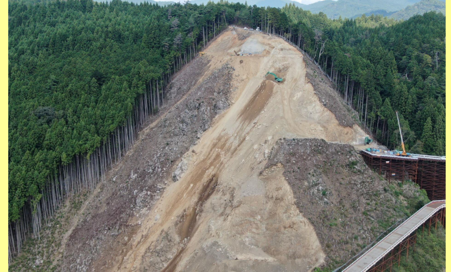
右岸掘削 (R6.9)
