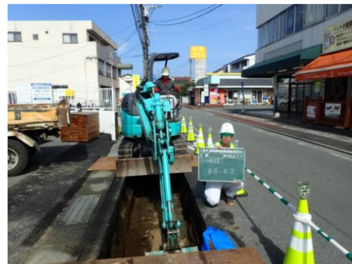
溝掘り部掘削
