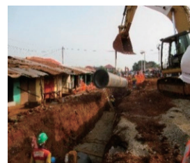
Installing ductile iron pipes (Completed in 2017)
