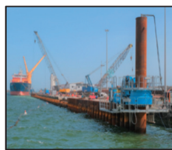
Rehabilitation of the quay wall of Dakar port in Senegal
