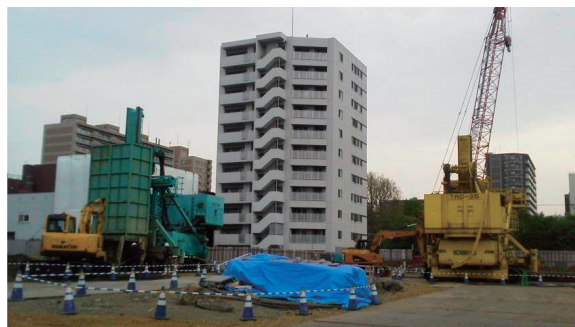
Diaphragm wall construction
