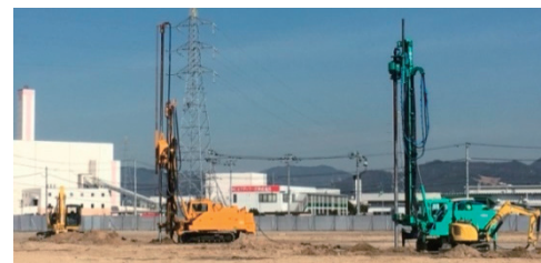
Construction scenery with 3SG Construction method
