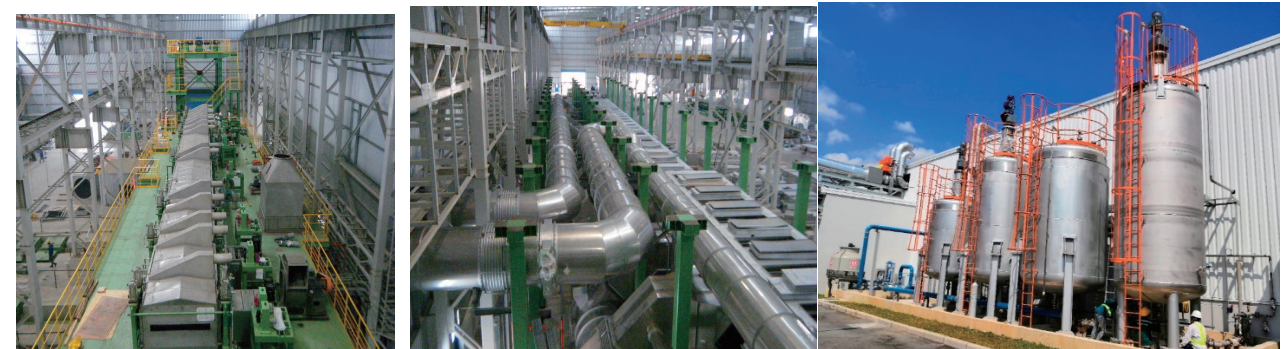
SOLTEC VIETNAM / SOLTEC HANOI – Fabrication (including Tank Design), Installation & Piping Works
