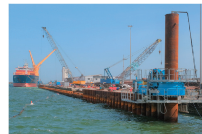
Construction without disrupting ship berthing or cargo handling (Senegal)
