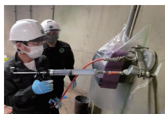
Crack injection work carried out at the Sao Paulo Luz Station Building (Brasilia)
