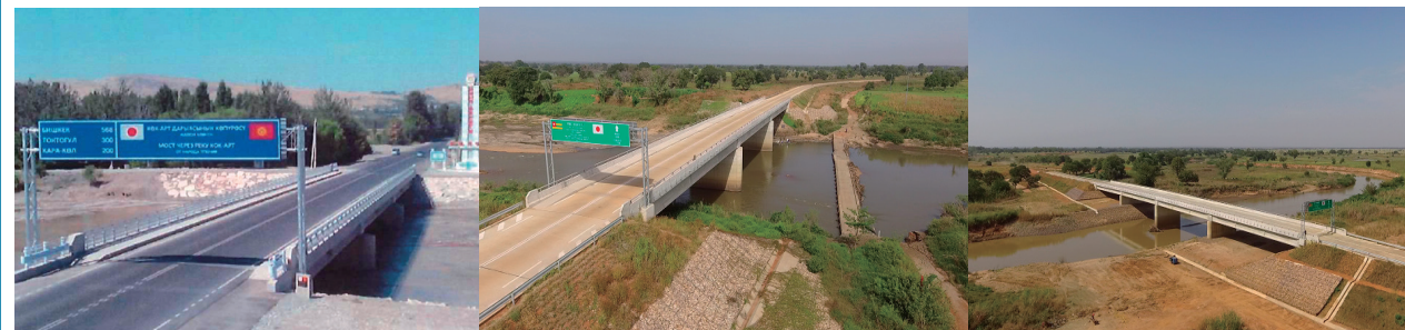
Project for Reconstruction of Kok-Art River Bridge on Bishkek-Osh Road in Kyrgyz
