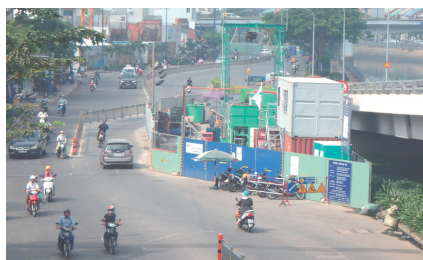
Showing construction site
