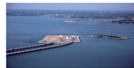
Hampton Roads Bridge-Tunnel
