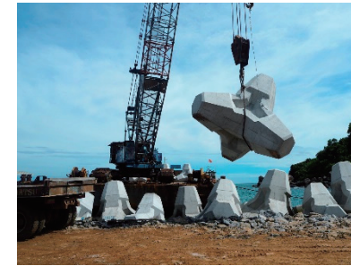
Breakwater for Chan May Port in Vietnam
