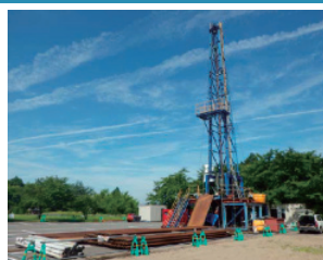
Site arrangement for well drilling (Hot spring drilling)
