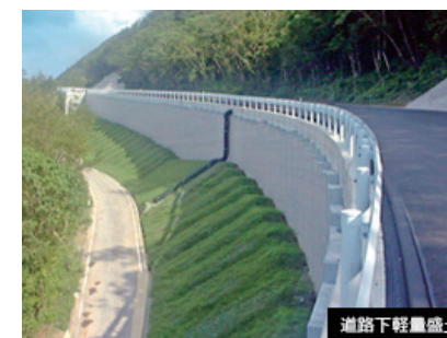
Road embankment (Japan)
