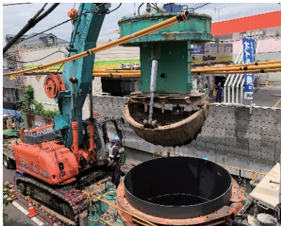
φ3000 standing pile
