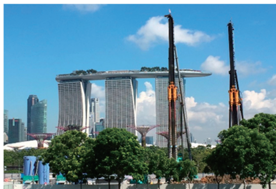
Singapore, Thomson East Coast Line T228 Project
