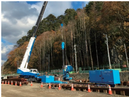
Disaster recovery (steel pile)
