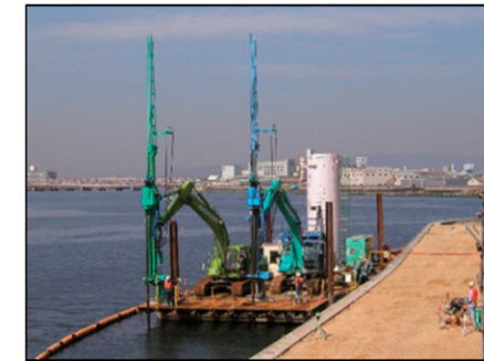
Construction from the barge
