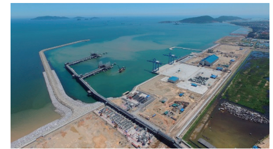
Breakwater for Nghi Son refinery in Vietnam
