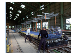
PC slab production
