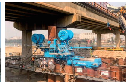
Bridge foundation construction with limited overhead clearance (Bangladesh)
