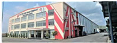
SOLTEC VIETNAM 1 st Factory
