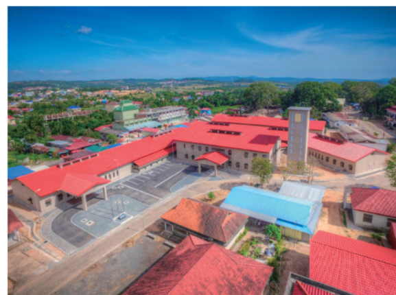
Overall View by Drone
