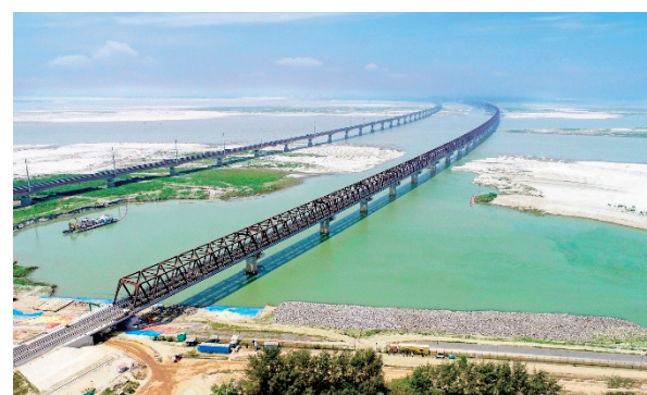
Figure 2. Example project delivery: Jamuna Railway Bridge, Bangladesh
