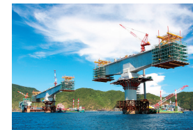
Cantilever erection
