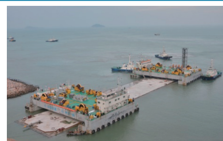
Hong-Kong Macao Connecting Bridge
