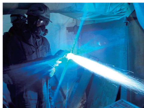
Figure 1. Anti-corrosion work using the TAPS method
