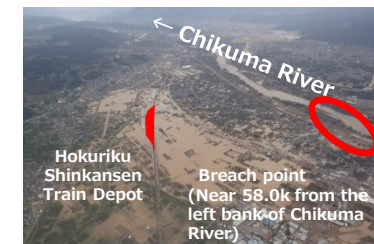
Flood damage caused by Typhoon No. 19 in 2019 (Chikuma River in the Shinano-gawa River system (Nagano City, Nagano Prefecture))
