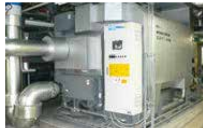
▲ 高効率吸収冷温水機 High Efficiency Absorption Water Cooling and Heating Machine.
