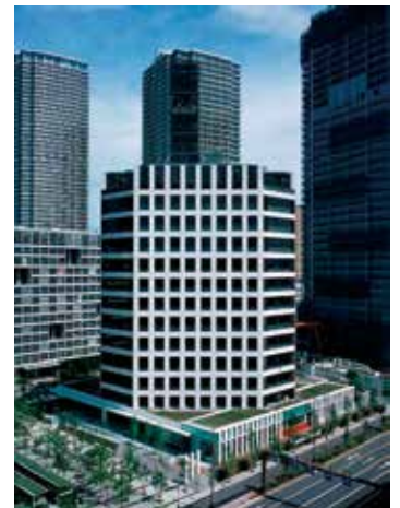
▲ 東雲合同庁舎 Shinjome Government Building
